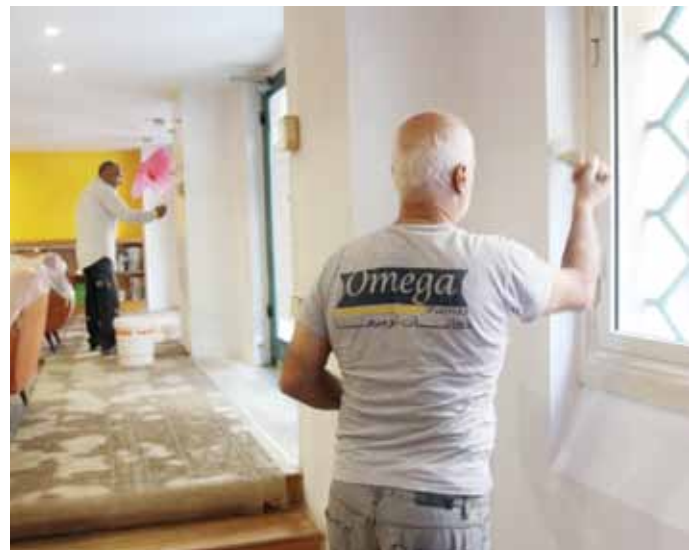
Al-Sabeel library renovation
