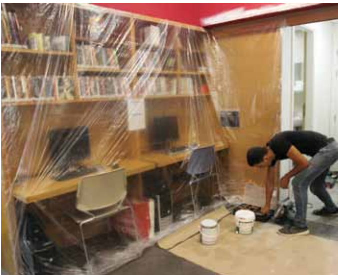
Al-Sabeel library renovation
