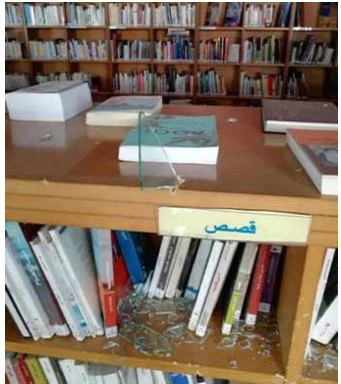
Al-Sabeel library renovation
